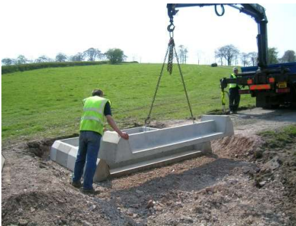
5. Allow base section spacing of 5mm
