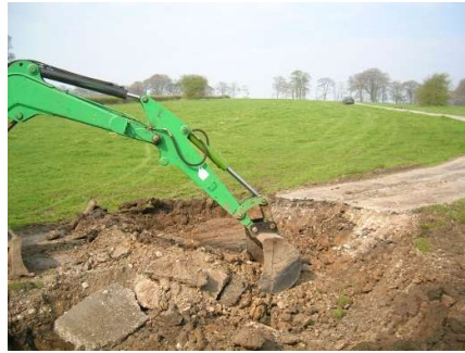
2. Excavate the pit. See the table on page 2 for dig dimensions
