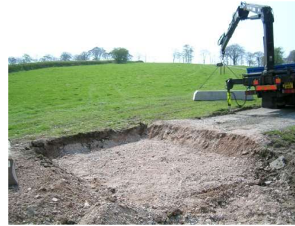
3. Prepare the base. As existing track or CBR test. (eg. 100-300mm of 0-40mm aggregate for sub-base)
