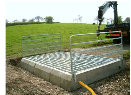
4. Use supplied cable loops to lift base sections. Check they are well screwed in before lifting
