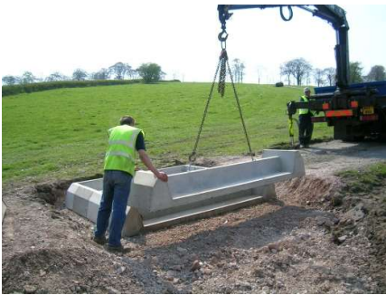
5. Allow base section spacing of 5mm
