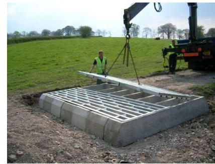
3. Prepare the base. As existing track or CBR test. (eg. 100-300mm of 0-40mm aggregate for sub-base)
