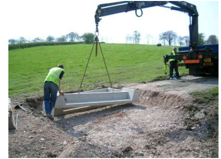
4. Use supplied cable loops to lift base sections. Check they are well screwed in before lifting
