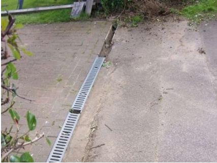
1. The Site Showing a typical installation; in this case replacing an inadequate slot drain.
