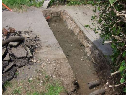
2. Excavate Pit and Prepare Sub-base Excavate to a depth of 750mm nominal. Eg. 300mm for the sub-base plus 150mm for the concrete bedding layer plus 300mm for the channel drain itself.
