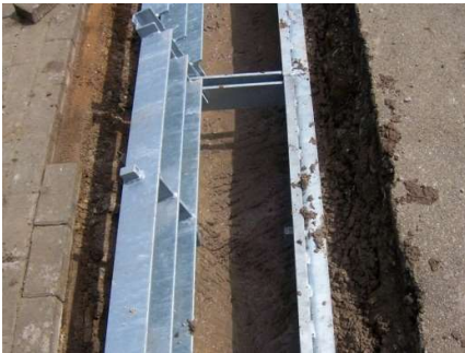
4. Stabilising the Units Bolt the units together and partially backfill with dry mix concrete to stabilise the units and to form the channel bed.
