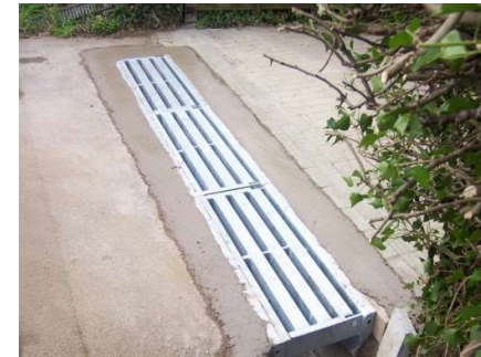
6. Installation Complete. NB. The outflow can run to either or both sides, or to a drain set in the base of the channel. In this case the outflow runs into a ditch.
