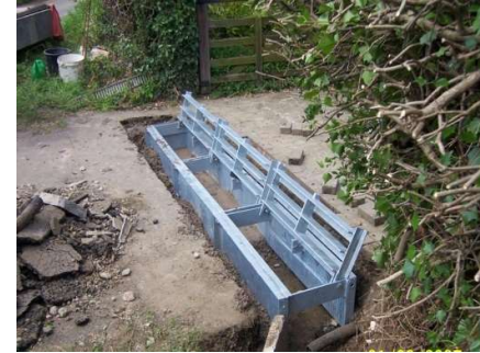
3. Bedding the Units In this case a dry mix has been used. The top of the units are set level with the road surface.
