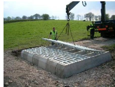
3. Prepare the base. As existing track or CBR test. (eg. 100-300mm of 0-40mm aggregate for sub-base).
