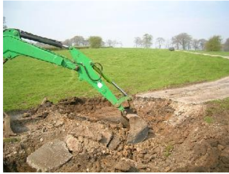
2. Excavate the pit. See the table on page 2 for dig dimensions
