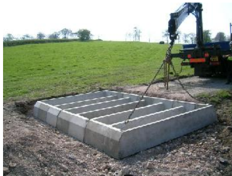
6. Drop in the grid sections ...
