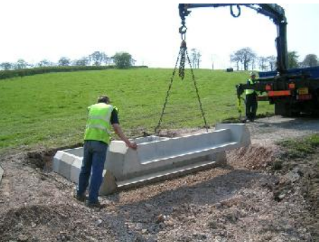
5. Allow base section spacing of 5mm.
