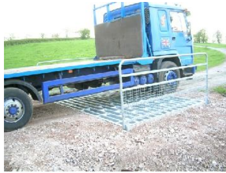
10. Job done ... completed in 4 hours.
